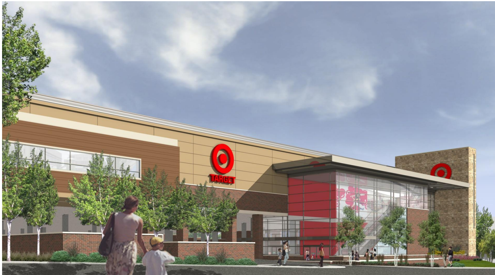
View to Main Lobby from Hilldale Way
